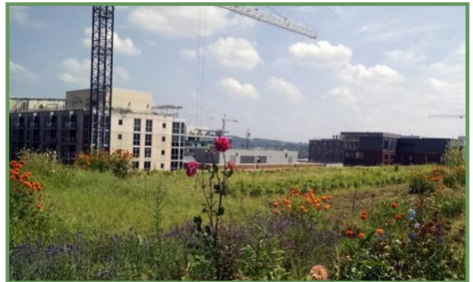
Figure 9: Flowers growing on a retro-fitted green roof at Up Top Acres in Washington, DC. Photo by Neith Little, UMD Extension.
