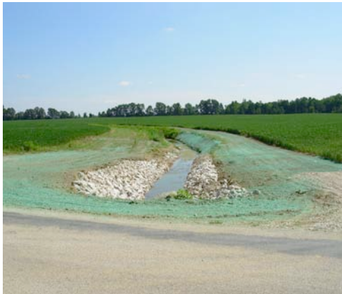
Left: Construction area stabilized by hydroseeding. Below, right: Inspecting seed germination at same site.
