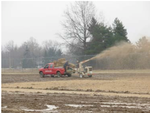
Above: Using strawblower to place straw mulch during winter.
